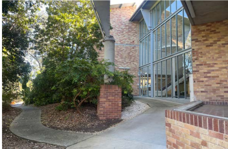
Main Entry A Block
