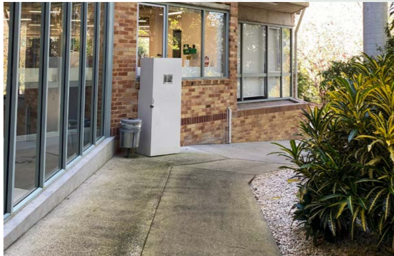
Entry Block A towards U Block
